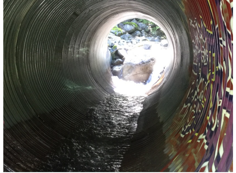
Looking through culvert from outlet
